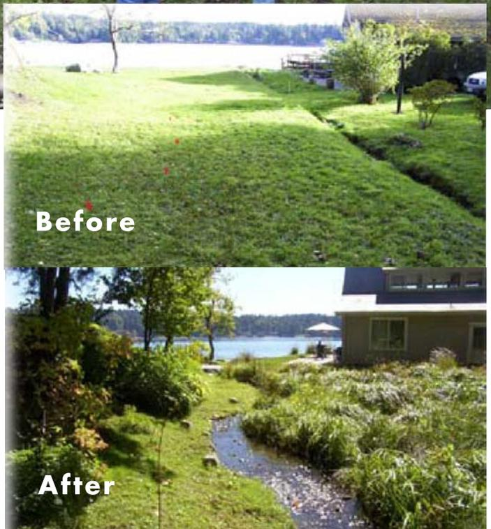
*These photos illustrate the relocation of a perennial stream into a naturally-configured channel. The channel was lined with erosion control fabric and the banks were seeded and planted with container-grown native species.*
